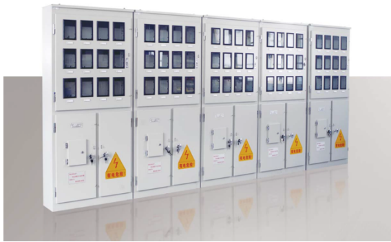
Epoxy Paint Spraying Paint
